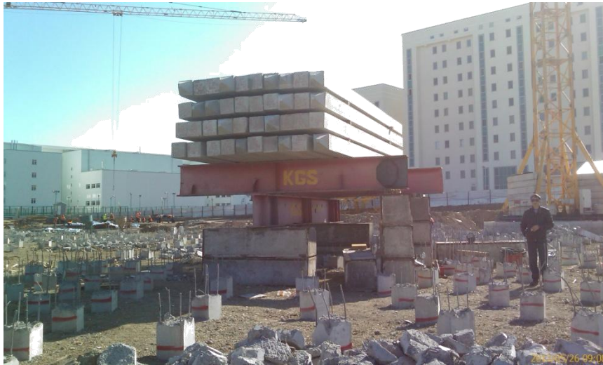
Figure 3. SLT for pile foundations of Nazarbayev University campus
