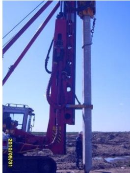
Figure 2. Test pile driving for DLT
