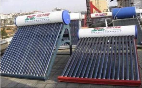
Fig. 2: Single-circuit solar water heaters
