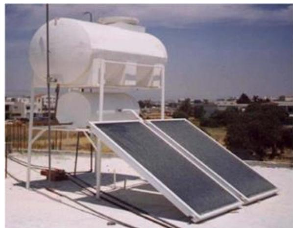
Fig. 1: Single-circuit solar water heater with thermosiphon
