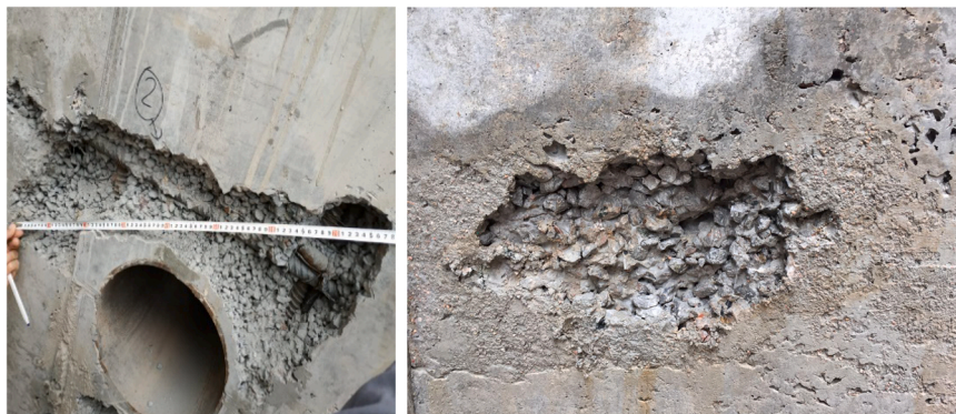
Fig. 1. Concrete failure during improper operation.
