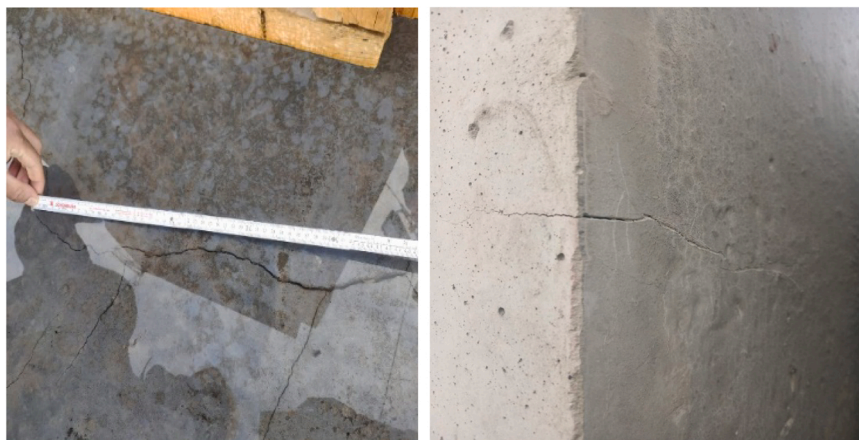
Fig. 2. Cracks as a result of concrete shrinkage in summer time.
