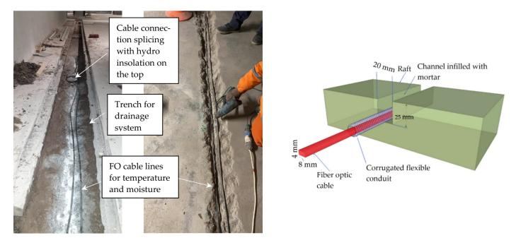
for cable integrity before any channels were infilled with cement mortar, allowing any breakages or localized losses arising from fiber damage to be rectified [13,16,17].
