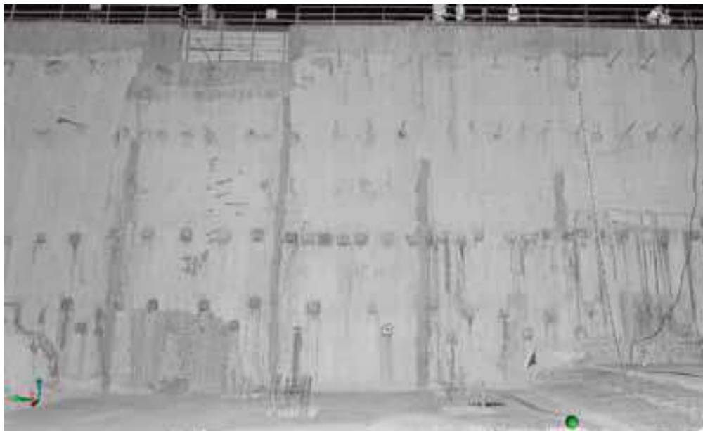
Figure 3: Image generated from the laser scanner illustrating the facade of the west section of the Dwall
