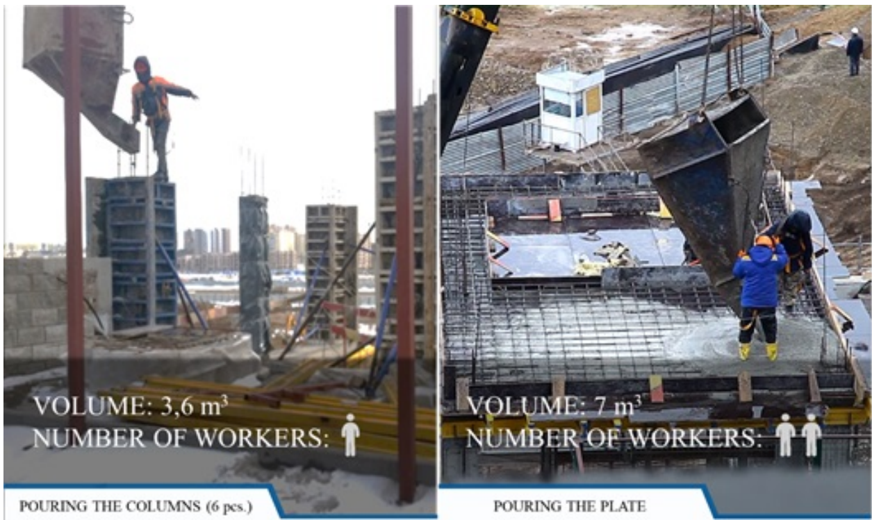
FIGURE 5 – Pouring SCC in the construction site of Green Quarter in Nur-Sultan
