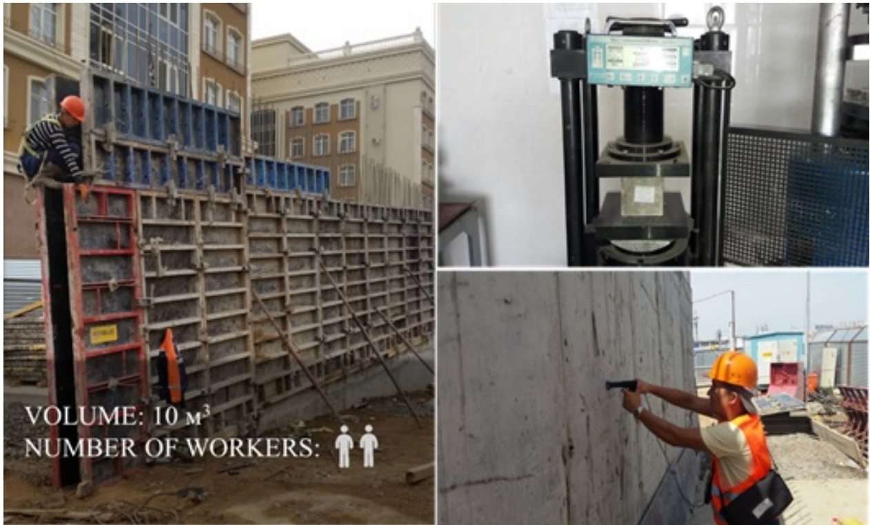
FIGURE 7 – Pouring SCC in the construction site of Sozvezdie in Nur-Sultan №1
