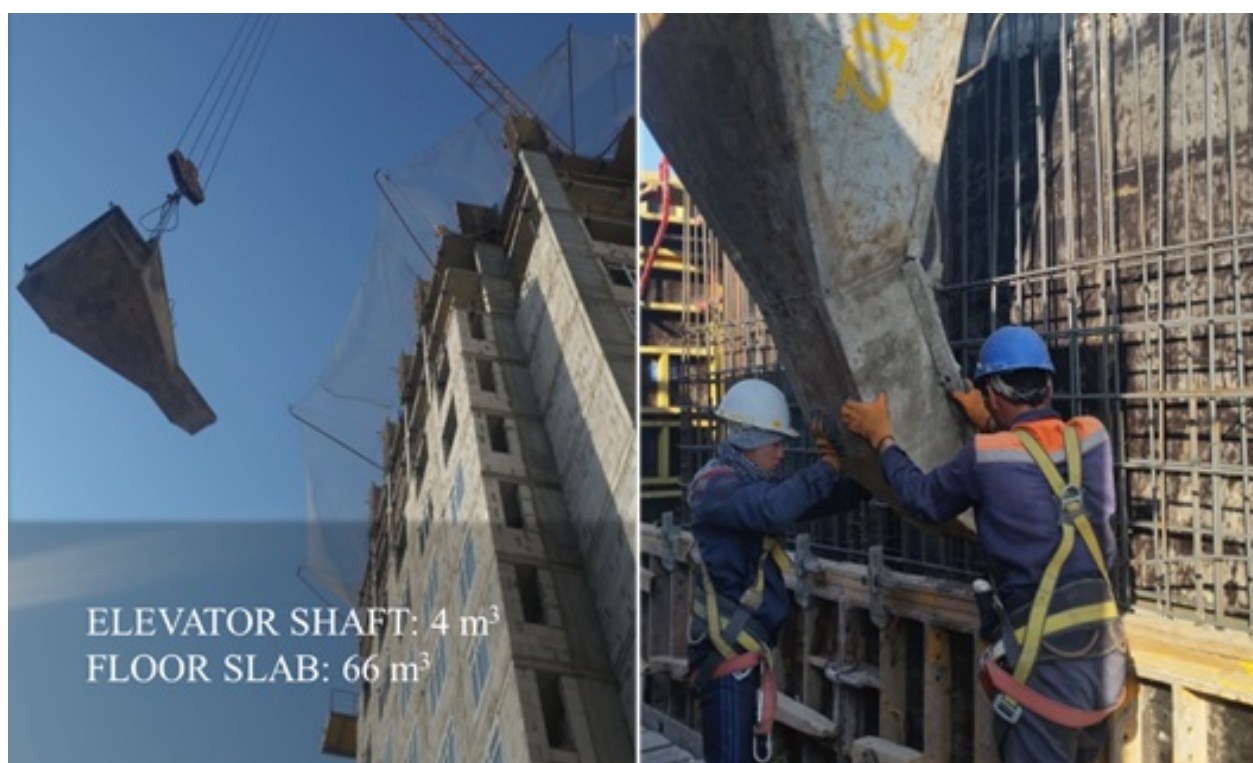
FIGURE 9 – Pouring SCC in the construction site of Sozvezdie in Nur-Sultan №2
