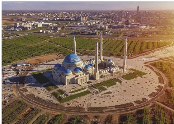
Figure 1. Construction site “New Mosque” in new Capital of Kazakhstan.
