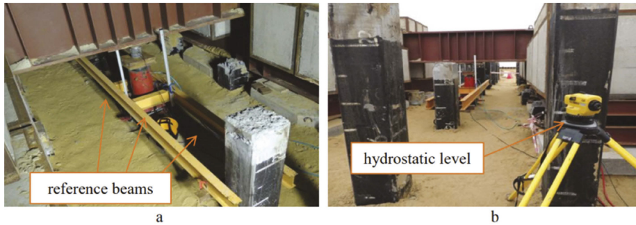
a - reference frame; b – checking the pile settlement with an optical level instrument
