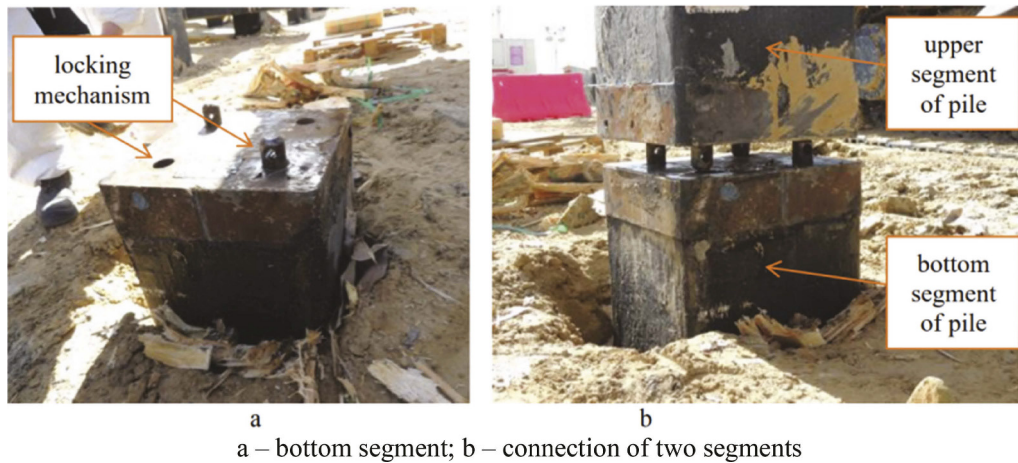
Figure 5. Two female (socket) and two male (stud) locking mechanisms.
