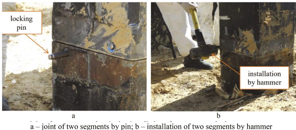
Figure 6. Installation of two segments of PCJP.
