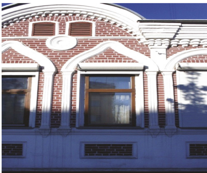
Figure 1. Crowned cornices with ribbon toothed brick brackets.
