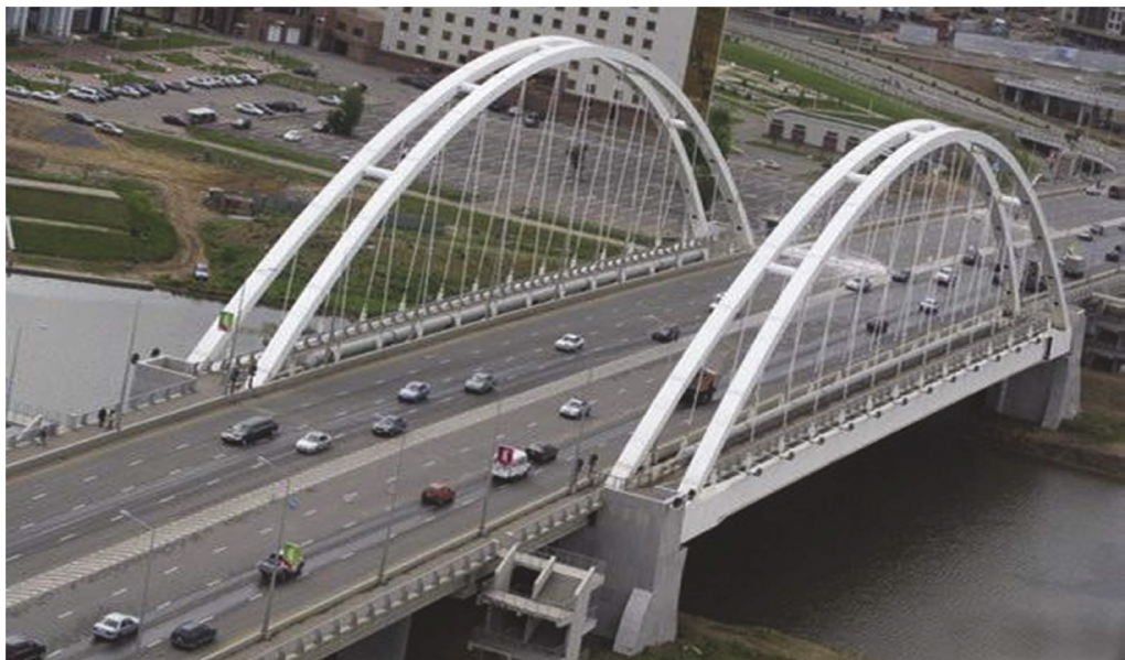
Figure 1. “Argali” bridge in Astana.
