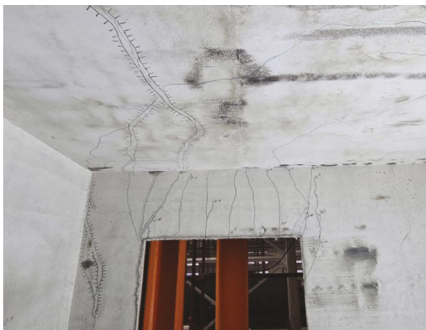
Figure 5. Damage to the interface between walls and ceiling slabs.
