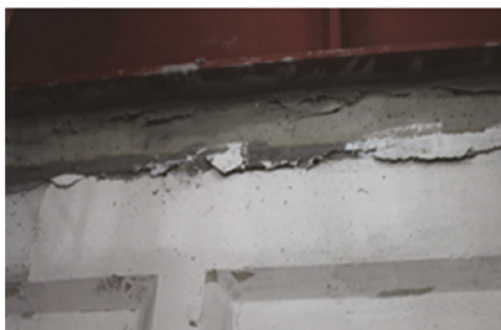
Figure 5. Damage to the interface between walls and ceiling slabs.
