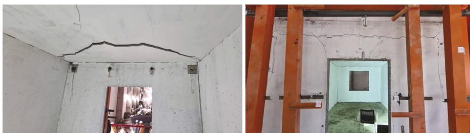
Figure 6. Splitting of the block floor slab No. 2.
