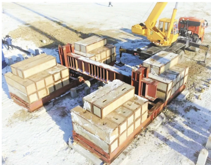
Figure 2. Assembling loads during mounting kentledge system.
