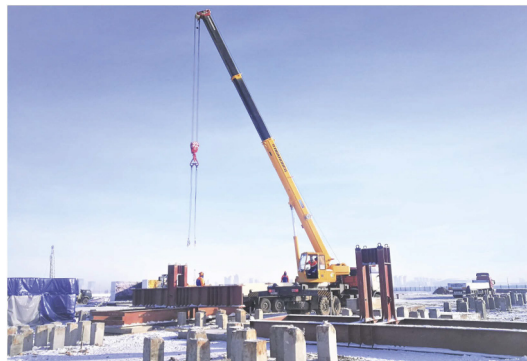
Figure 1. Mounting kentledge system.
