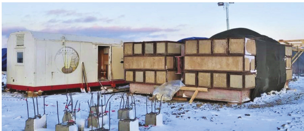
Figure 4. General view of the kentledge system with a container for test.
