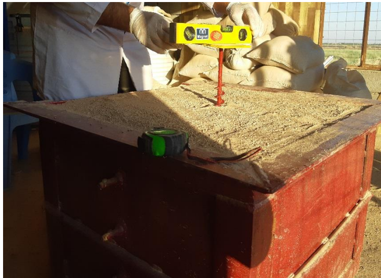
Figure 4. Installation of screw pie in the steel box container.
