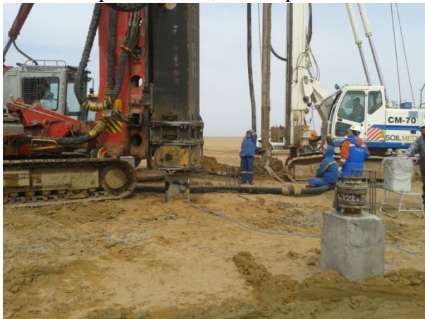
PDA and dynamic load test
