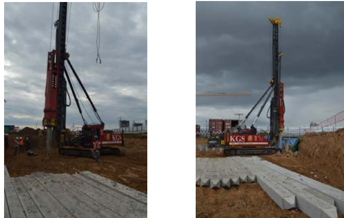
Figure 2. DLT of piles using driving machine Junttan PM-25
