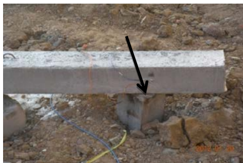
Figure 3. Preparation of the piles for the PDA
