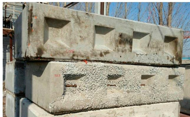
**Figure 11.** The upper product is made of SCC with silica fume, while below it, for comparison, is an identical product made of conventional concrete of the same strength class, produced without vibration compaction.
