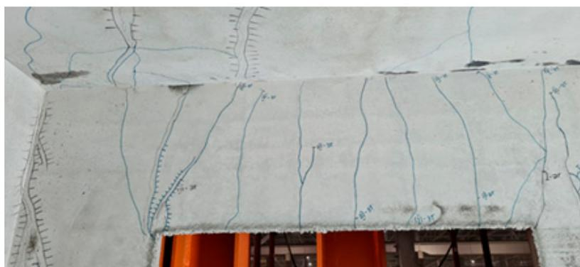
**Figure 22.** Damage to the lintel above the doorway of the longitudinal wall doorway.
